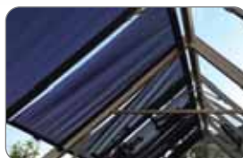
Internal roller blinds for roof or side
