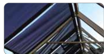
Internal roller blinds for roof or side
