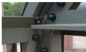
Strong Frame with box section glazing bars
