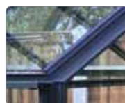
Screw-in bar capping system
